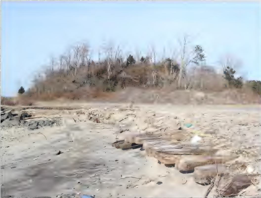
Figure 4.4. View looking northwest at Battery Kingman. South of Battery Kingman, coastal erosion has exposed wooden railroad ties. The ties are remnants of a railroad system that delivered ammunition to the coastal defense batteries throughout Sandy Hook. After this picture was taken, continuing coastal erosion completely removed the railroad ties (Olmsted Center, January 2009).
